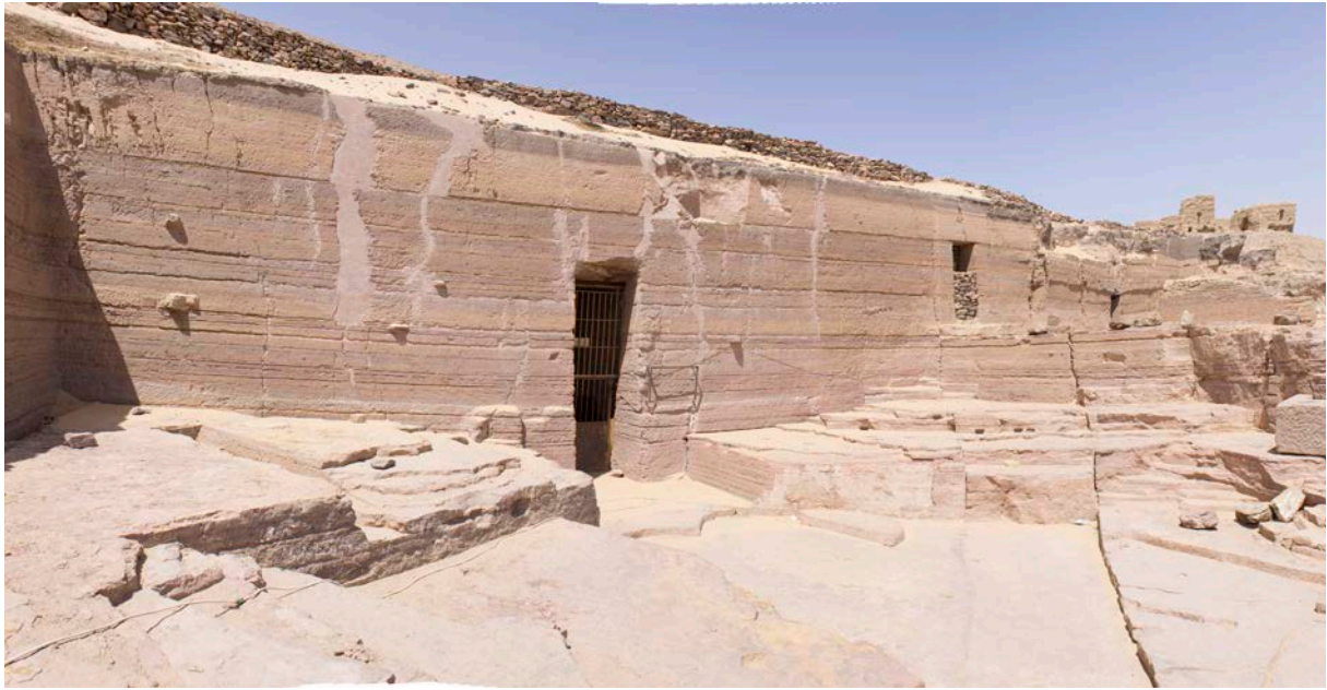
Fig. 8. To the right is a crack that crosses the courtyard of QH31 and continues, in the background, onto the façade of QH33. Photograph by Fernando Martínez Hermoso (2014 campaign).
