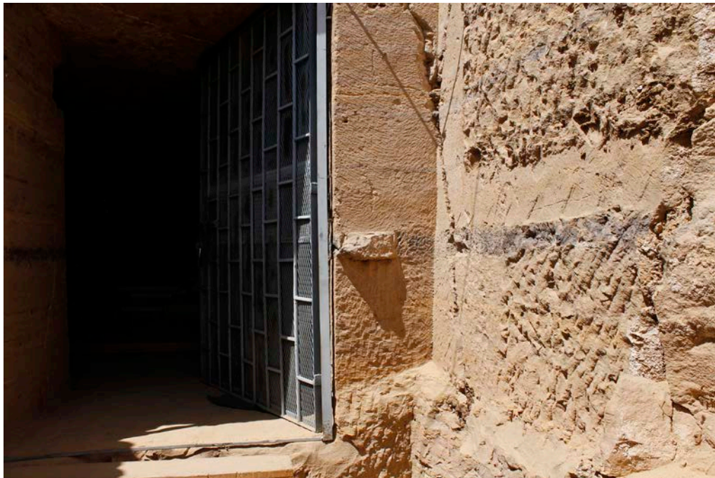
Fig. 13. Detail of a finished strip of 10 cm in the façade walls and side walls of QH33. Later, the QH34 tomb was excavated and its barrel-vaulted adobe corridor was built. Photograph by Fernando Martínez Hermoso (2014 campaign).
